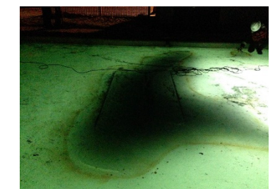
Oil trapped in cavities highlighted with underwater lights and cameras.
