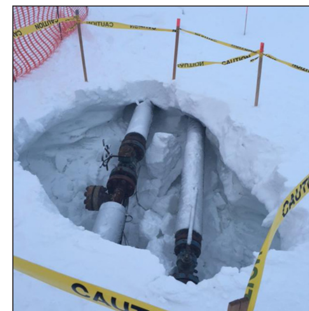
Snow-covered flowlines may create thaw pockets that can cave in under the weight of personnel.
